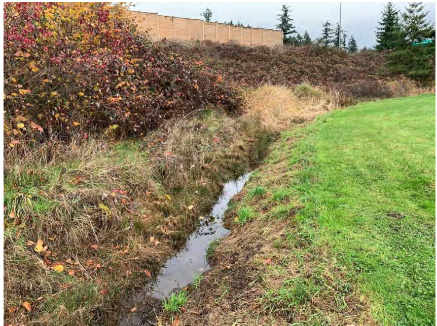
Photo 2. Drainage ditch on north boundary to be converted to vegetated swale.
