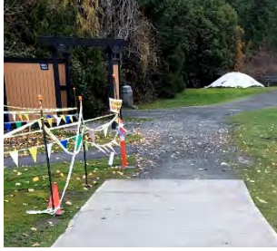
Hazardous situation where concrete meets granular at bottom of slope
